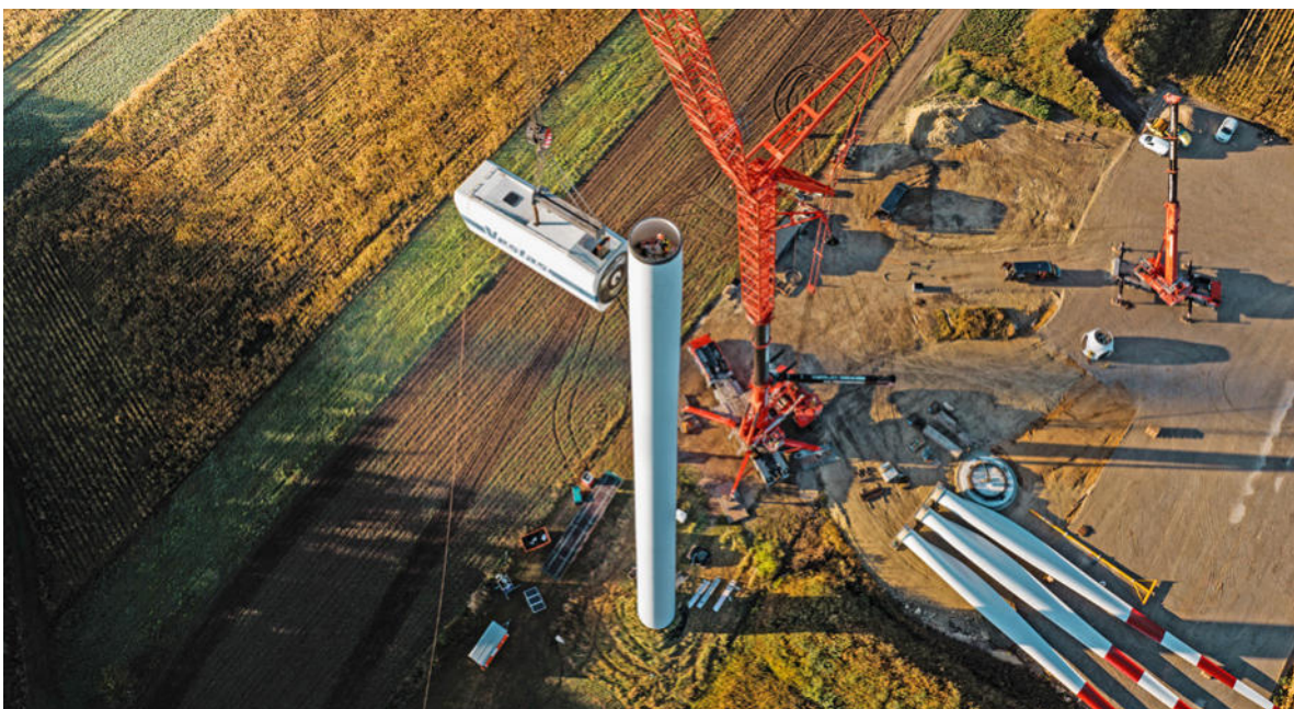
The turbines were carefully dismantled because they are set to be reassembled and used again at another site.
