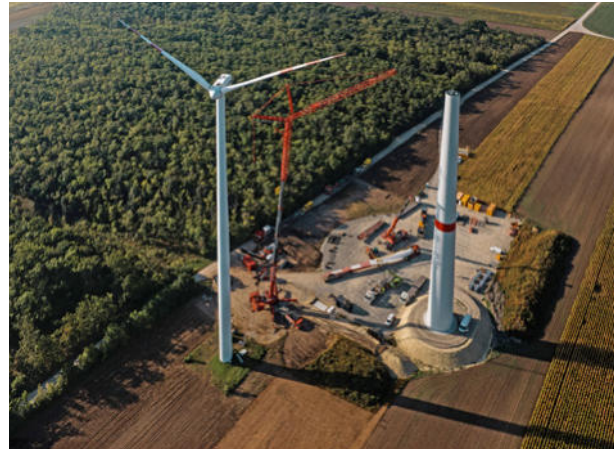
Dismantling of the old turbines begins as the new turbines are erected.
