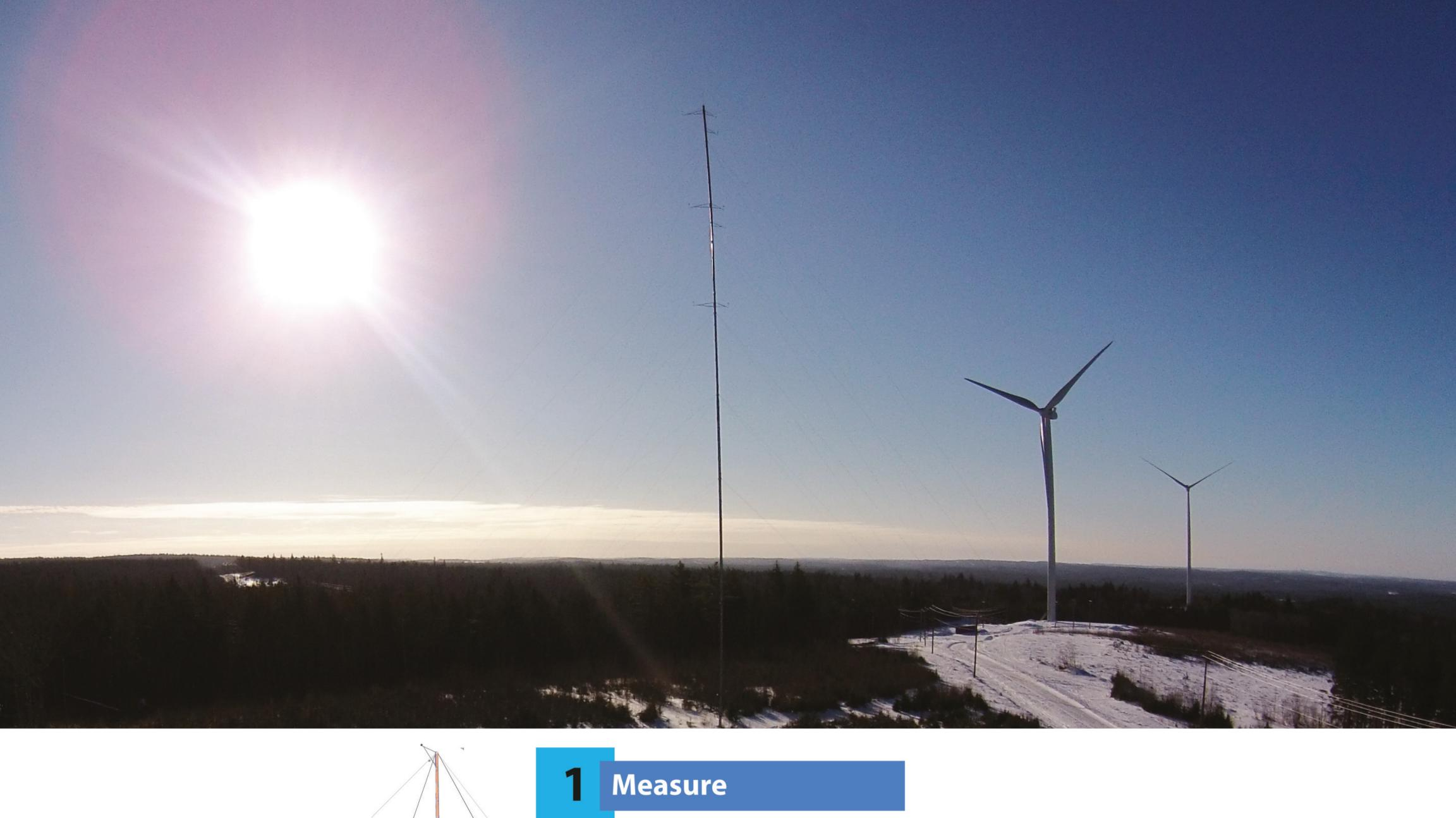
Meteorological test towers measure the wind speed, temperature, humidity, and barometric pressure over a full year.
